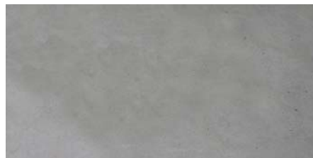
Cementitious / structural overlay
