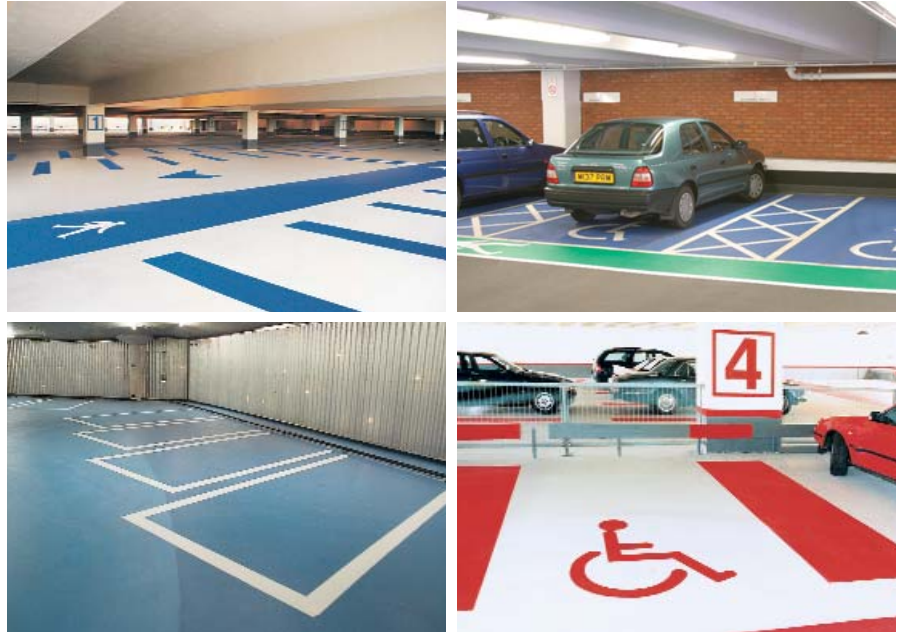
Heavy duty, thick layer, waterproofing and surfacing system for internal car park decks
