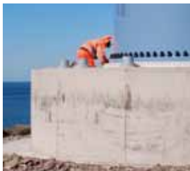
4 Preparation of the substrate by means of abrasion.
