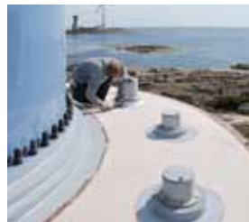
8 Waterproofing of the connections with Triflex Towersafe.
