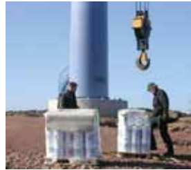
2 Loading with the deck crane.
