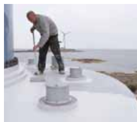
11 The finish is finally applied ...
