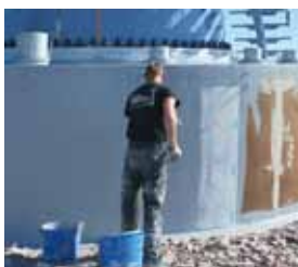
10 ... waterproofed with Triflex Towersafe.
