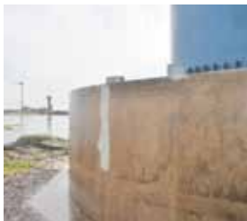
7 ... and surfaces with Triflex Towersafe Primer.
