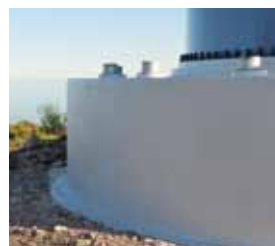
12 ... using Triflex Towersafe Finish.
