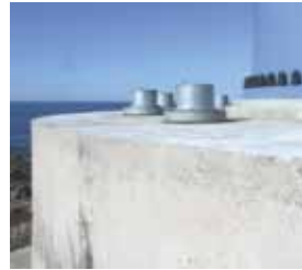
3 Naturally weathered foundations.
