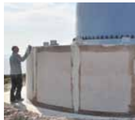
5 Levelling off of the formwork edges with Triflex Towersafe Paste.
