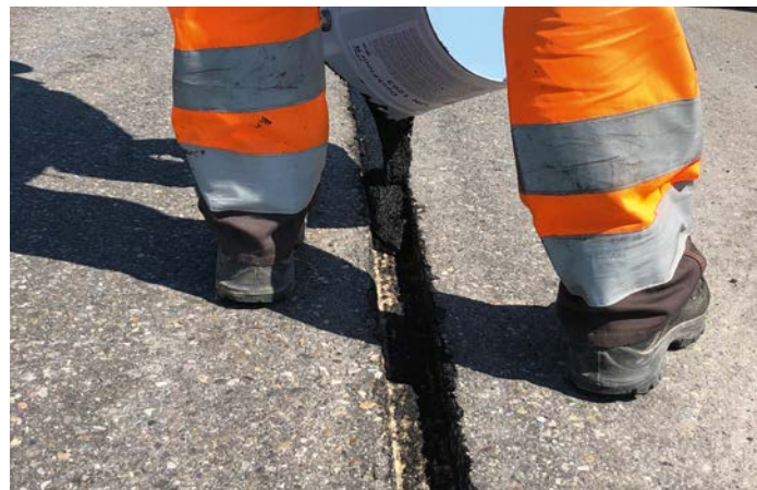
Repair of split asphalt day joint to roundabout.
