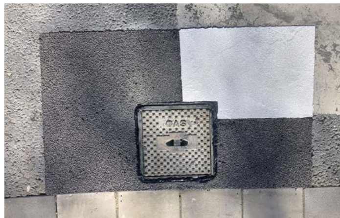
Repair of asphalt to perimeter of gas inspection cover
