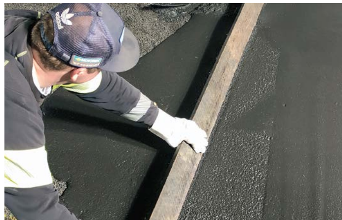
New road construction – levelling of subsidence.
