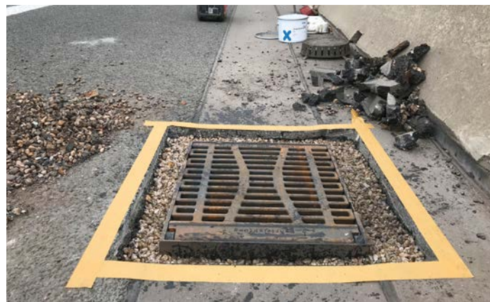
Perimeter fixing of bridge drainage outlet frames
