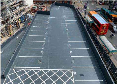
Originally the client looked to remove the asphalt and replace with a new asphalt covering. However, Triflex working with Triflex Authorised Contractor CRL, proposed a system that could overlay the existing asphalted surface. By leaving the asphalt in situ, the programme of works was shortened and the structure could be waterproofed with minimal disruption. Located in the city centre, this meant the hassles of removing large amounts of asphalt and its transport away was avoided.
