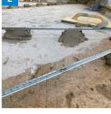
Complete to a smooth finish: Continue to smooth and level rough areas in the surface, with additional application of small amounts of Triflex Cefix Screed 631. Continue to smooth with PU float until uniform.
