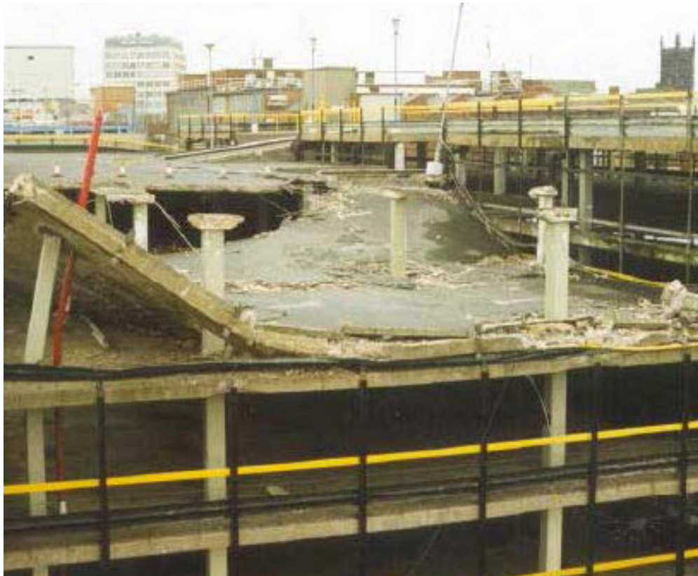
Pipers Row car park, Wolverhampton in 1997. Partial collapse attributed to carbonation and a lack of waterproofing to cracks: https://www.hse.gov.uk/research/misclindex.htm
